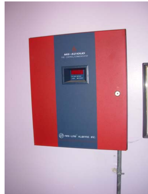
20. Fire detection - monitoring panel, located in front foyer
