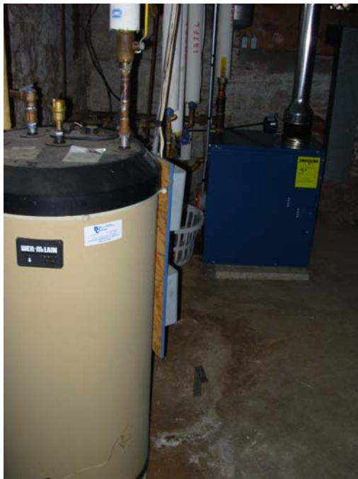
19. Heating and DHW equipment in basement
