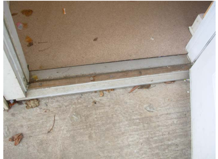
8. Door threshold modifications needed at accessible entrance
