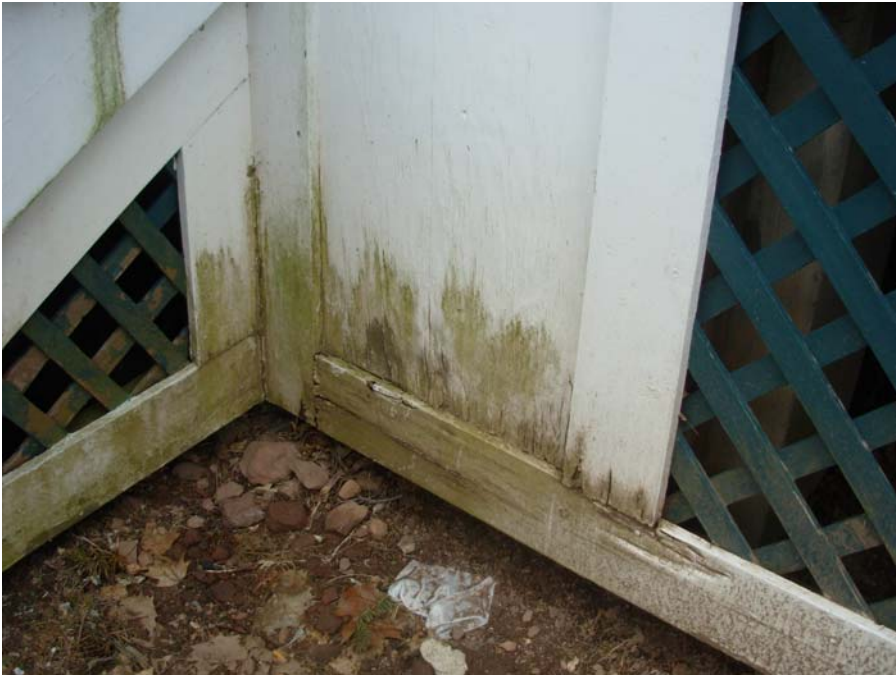
5. Wood deterioration at front porch
