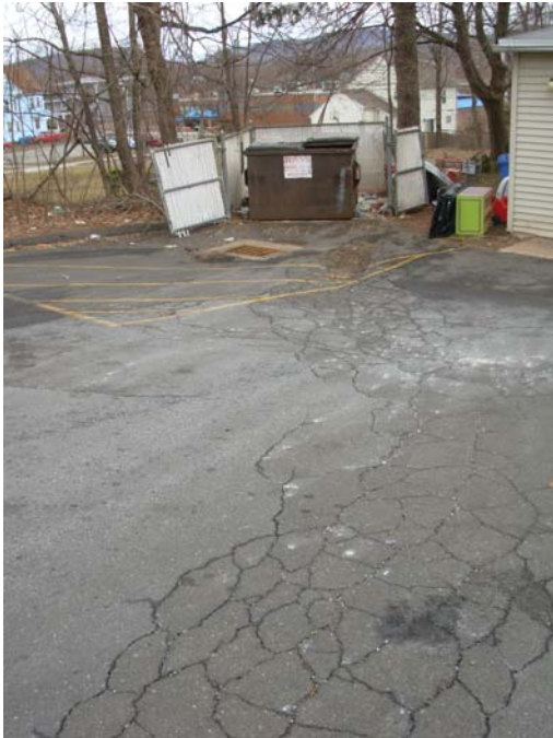
1. Deteriorating and settling paving at parking lot
