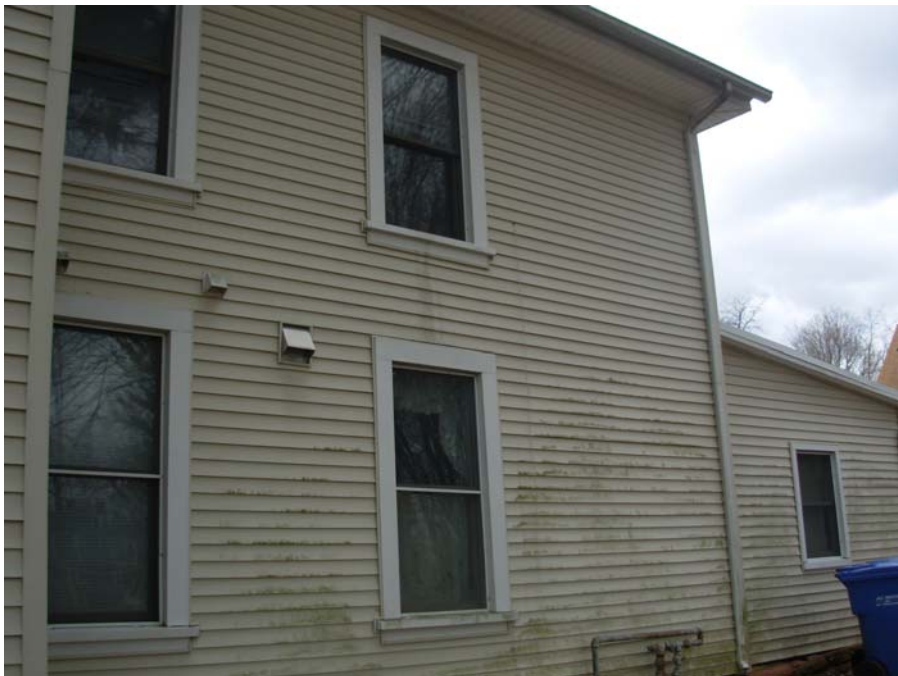
3. Minimal damage and organic material growth at vinyl siding
