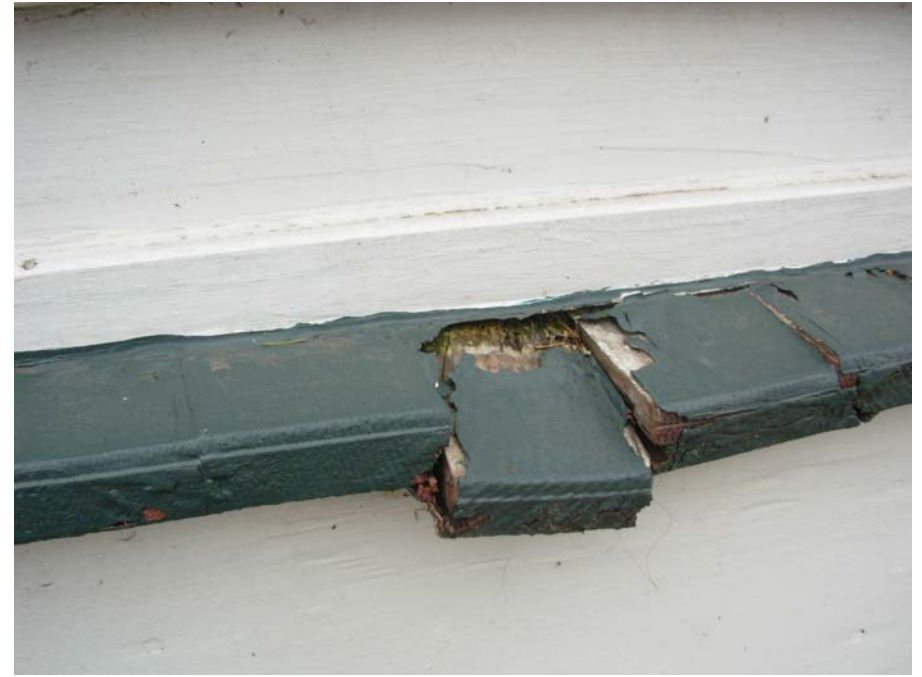
6. Decking and column base deterioration at front porch
