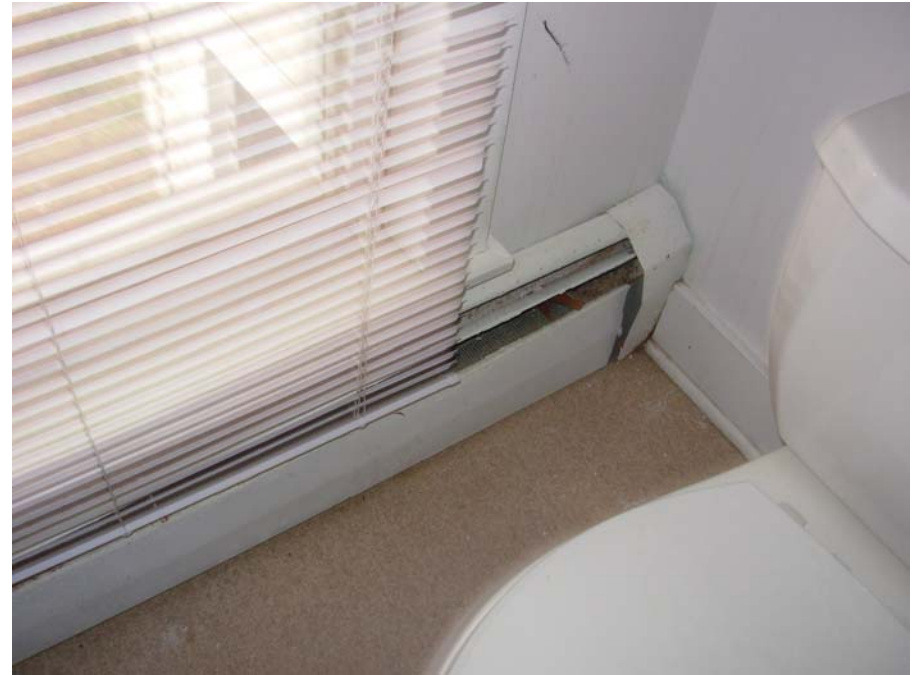
18. Damaged radiators and covers in most rooms
